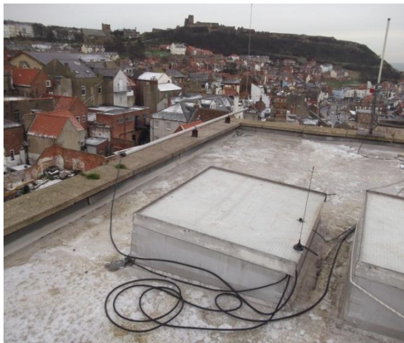
Antenna location and coaxial cable run through skylight
