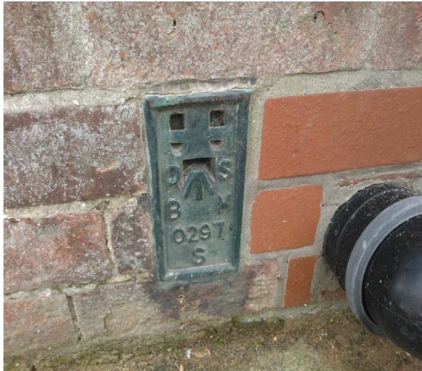
Port benchmark used to level in tide gauge
